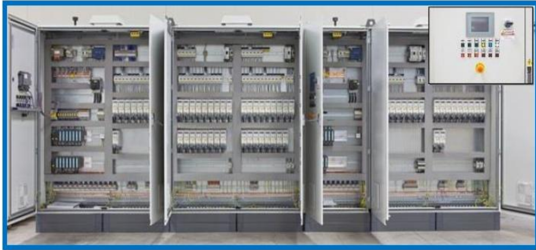
Electrical control cabinet for line automation
